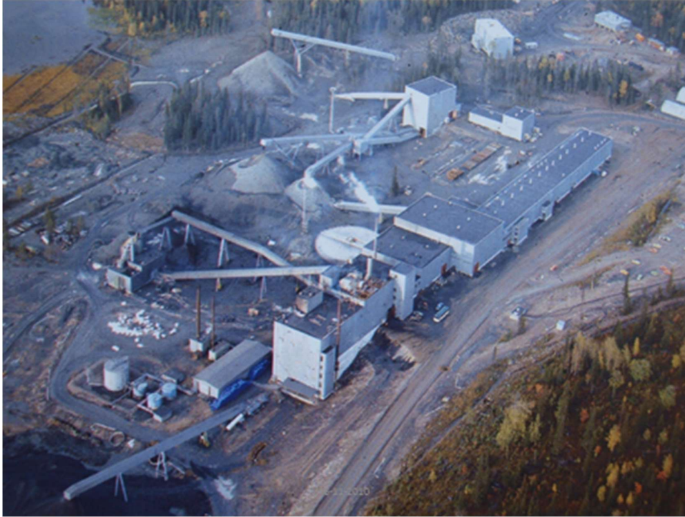
Figure 6-1 Aerial photo from Rautaruukki processing plant in 1976.
