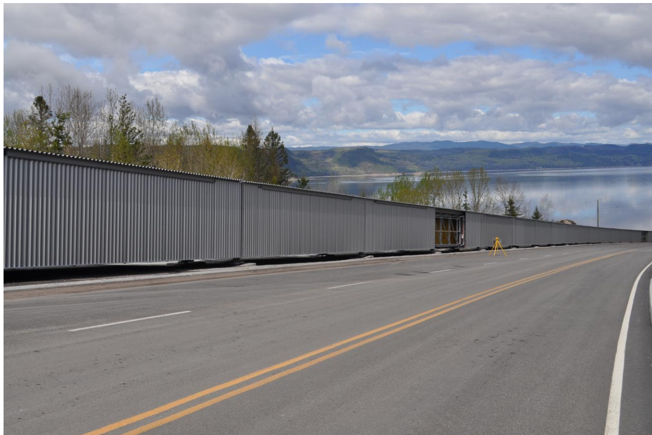
Figure 1: Installed pipe conveyor modules between the wharf and planned site for the 4Mt iron pelletizer plant.
